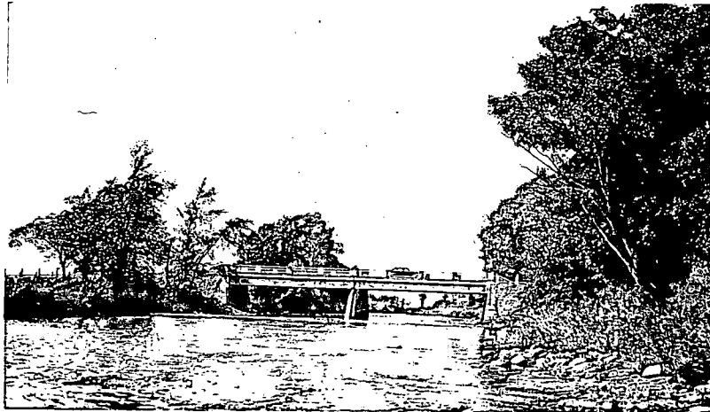
BRIDGE OVER BULLSTRODE RIVER AT HALIFAX NORD, (STE-SOPHIE), MEGANTIC COUNTY. (STE-SOPHIE-PRINCEVILLE HIGHWAY).- Two spans forming a total length of 103 ft. 6 in. Reinforced concrete beams and slab on concrete substructure. Width of roadway 24 ft. Built in 1936.
