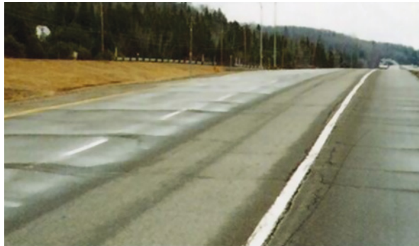
Figure 13 Fissures transversales
