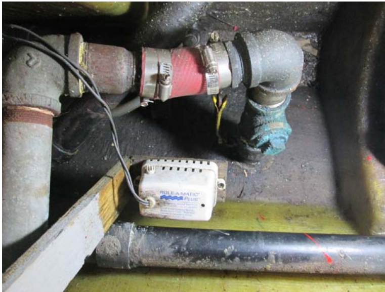
Photograph 18 - Salt water intake, engine room forward
