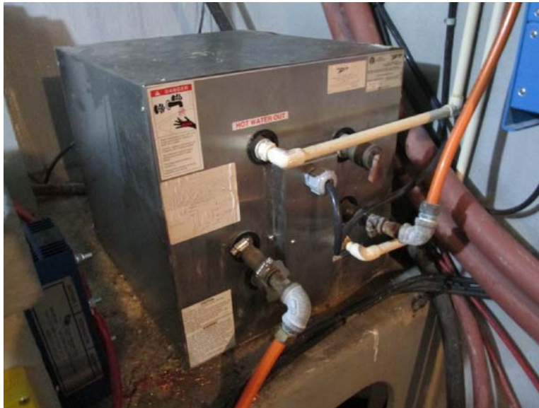
Photograph 21 - Domestic water heater
