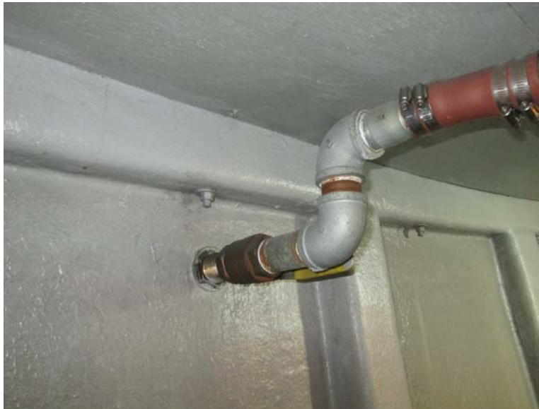
Photograph 23 - Typical through hull discharge (salt water)
